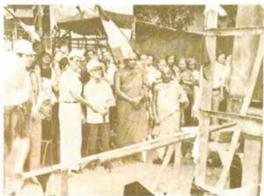
First pile for building Extension
