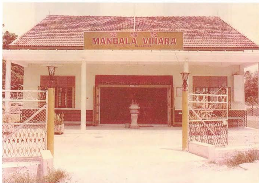
The original building of Mangala Vihara
