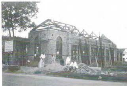
Outram Road Vihara: Nearing construction
