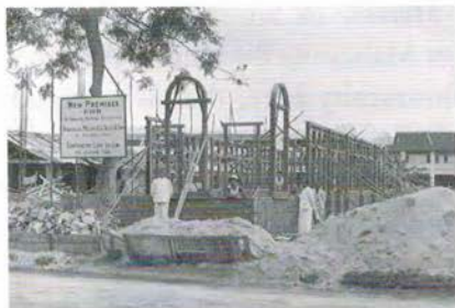
Outram Road Vihara: Under construction
